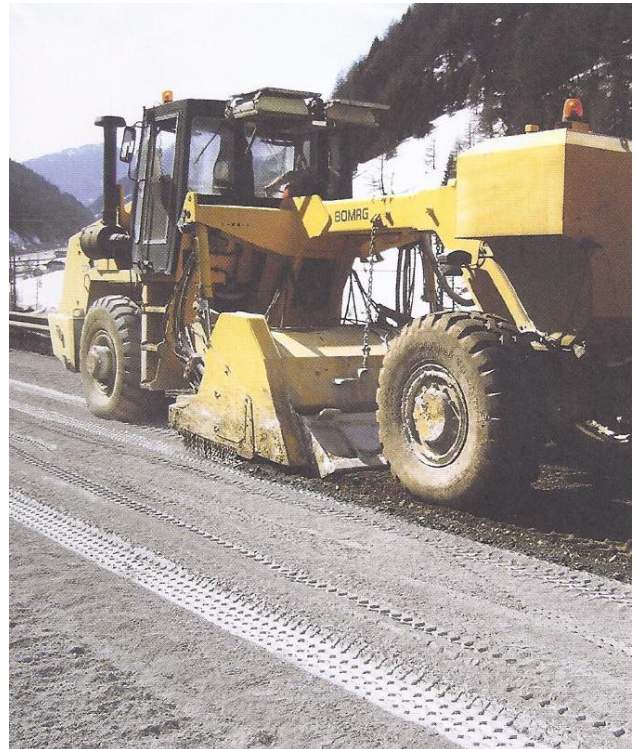
Figure 2 – Cold recycling of base course
