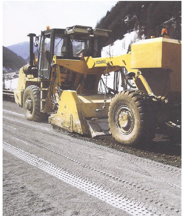
Figure 2 – Cold recycling of base course
