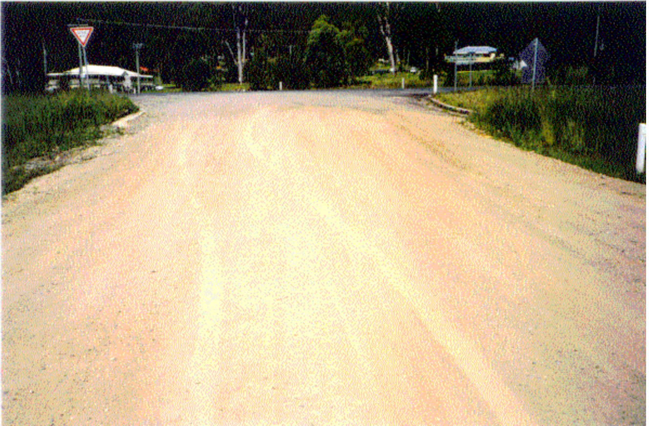
Photo 16 Renolith - cement treated sand pavement section of Wonglepong Road after 28 days.
