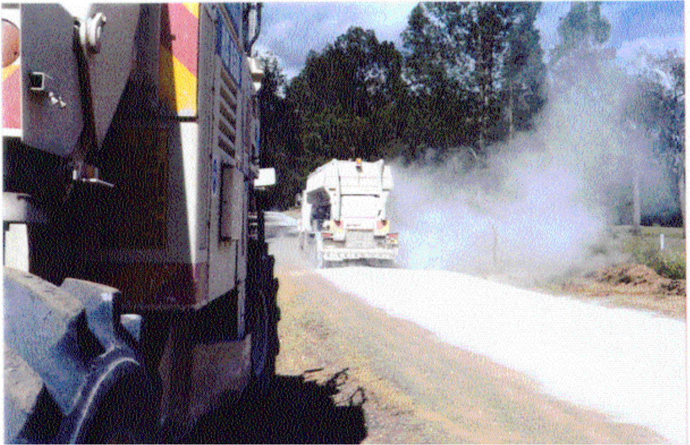
Photo 1 Cement spread over existing pavement material of Wonglepong Road.
