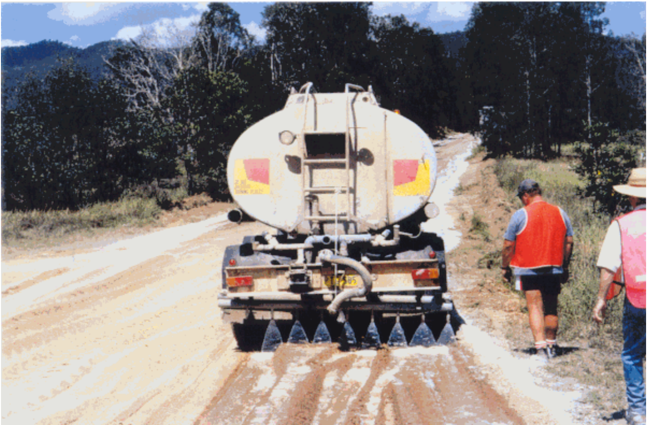
Photo 3 Water truck spraying Renolith / water onto mixed cement pavement material.
