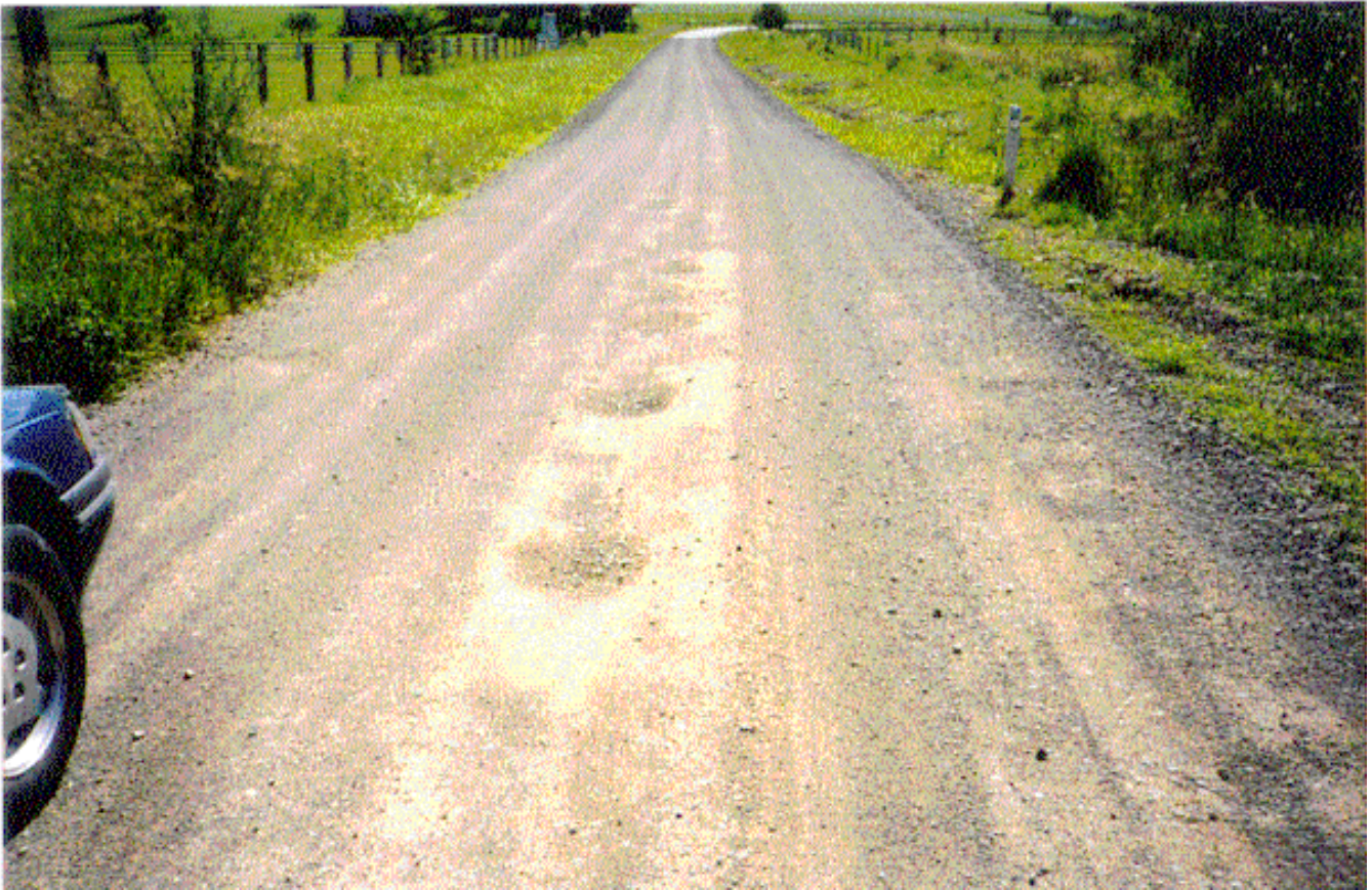
Photo 13 Wonglepong Road existing pavement after maintenance grading. Note high level of loose gravel on surface.
