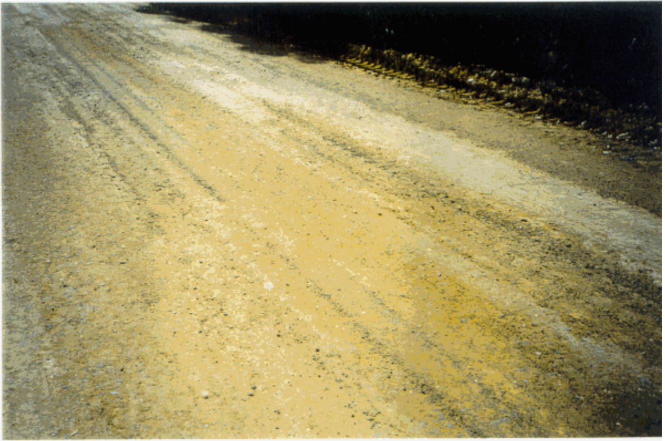
Photo 8 Renolith - cement treated orange sandy clay pavement material.
