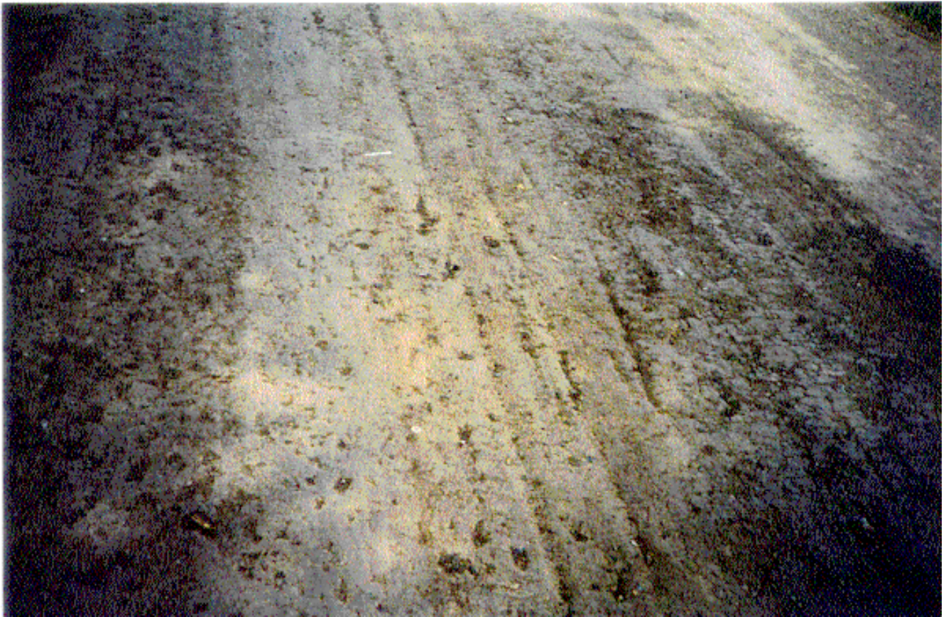
Photo 12 Renolith - cement treated sandy clay soil / gravel pavement material.
