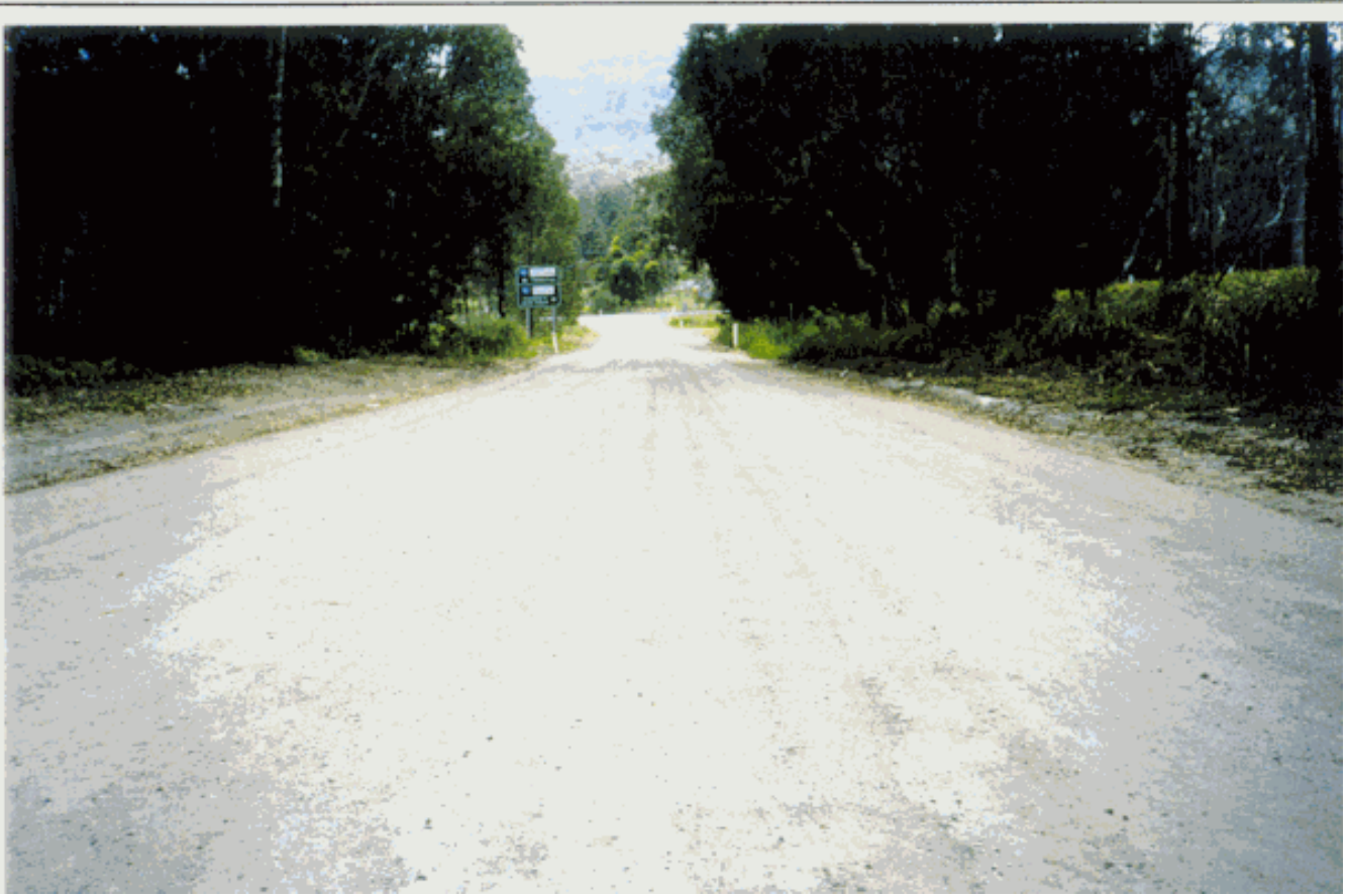
Photo 5 Renolith - cement treated sand pavement section of Wonglepong Road after 7 days.
