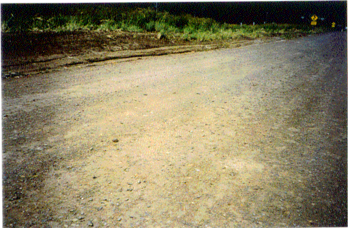
Photo 10 Renolith - cement treated black soil pavement material.
