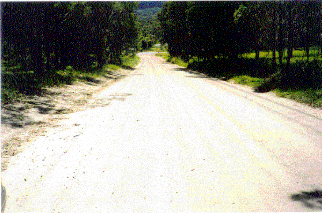
Photo 15 Renolith - cement treated sand pavement section of Wonglepong Road after 28 days.
